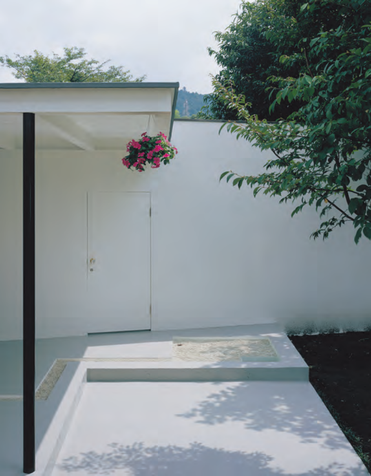
Spring Water Pavilion (2004) near Mount Fuji, welcomes spring water in to flow through a concrete channel, cooling the floor in the hotter months. Image: TANK Co., Ltd and Kozo Takayama.
